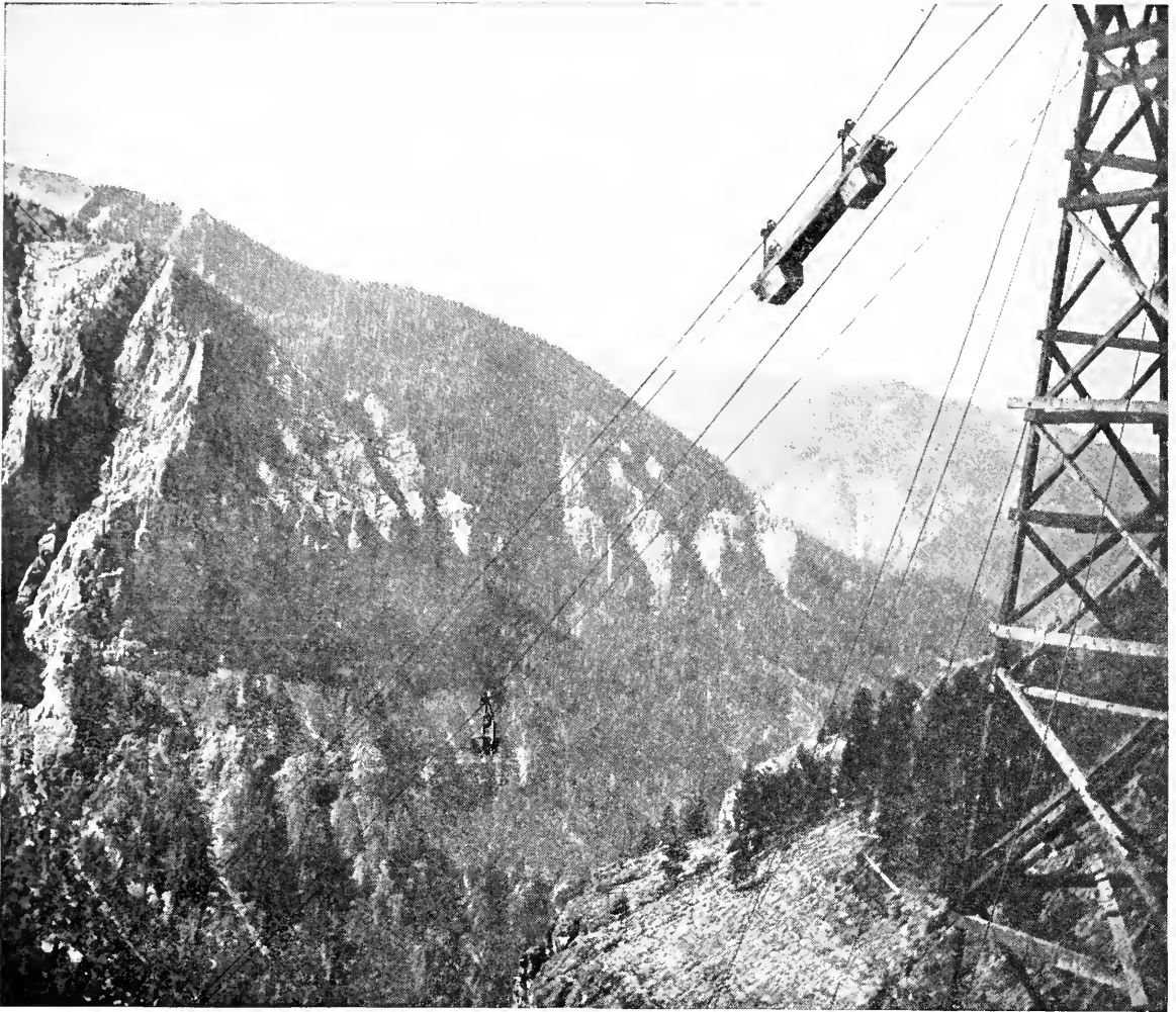
CABLING LUMBER ACROSS A CANYON
